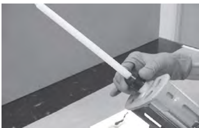
Attach static mix tip to cartridge
