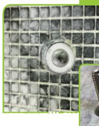
Completed installation. For undermount sink applications, a threaded post, sink clip and wing nut may be applied during countertop installation. Properly installed KEEP-NUT™ can support up to 562lbs per anchor\*.
