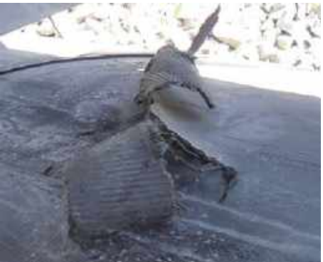
Before: R-Flex® Repair
