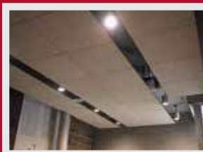
Panel and Ceiling Hanging
