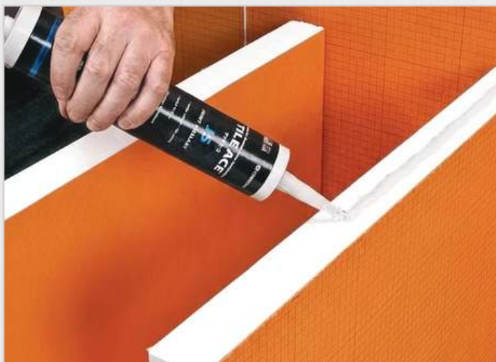
Sealing Seams and Fastener Penetrations in Foam Backer Board
