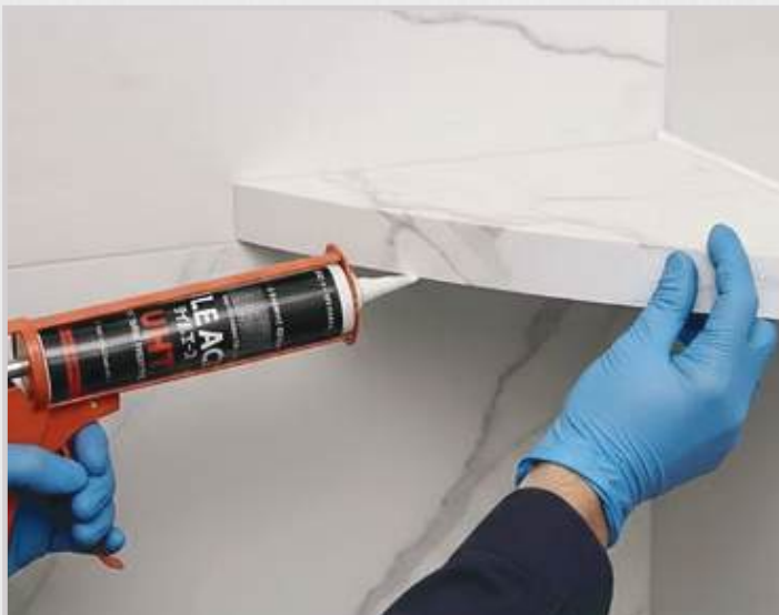
Applying Large Format Tile to Honeycomb Panel Backer Board
