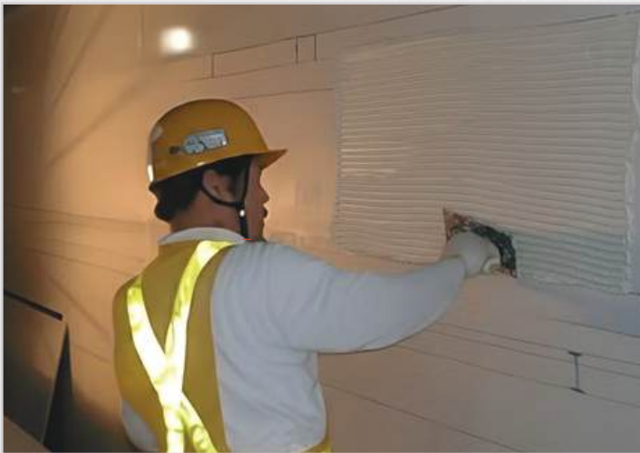
Direct to Wall with Notched Trowel
