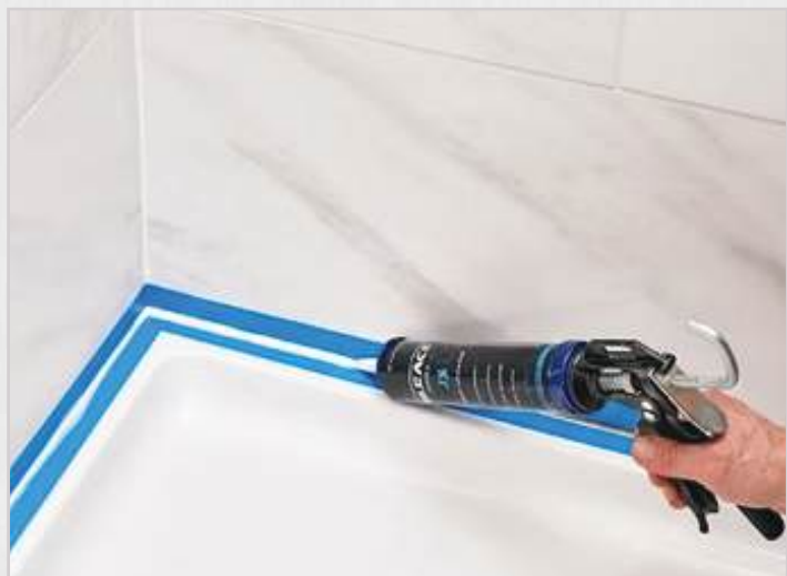
Waterproofing Transitions and Tub Flanges After Tile Installation
