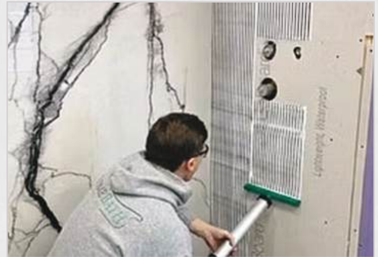
Direct to Wall with Sausage Gun and MaxSpreader Nozzle
