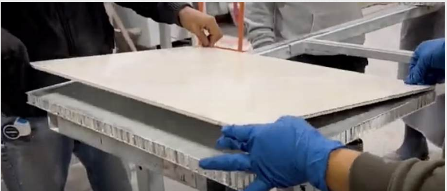
Applying Large Format Tile to Honeycomb Panel Backer Board
